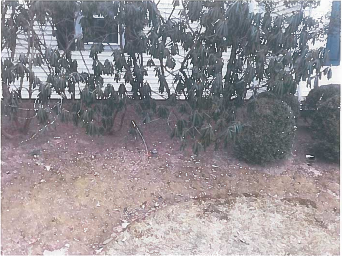
Photograph 1: 550 gallon UST in ground
