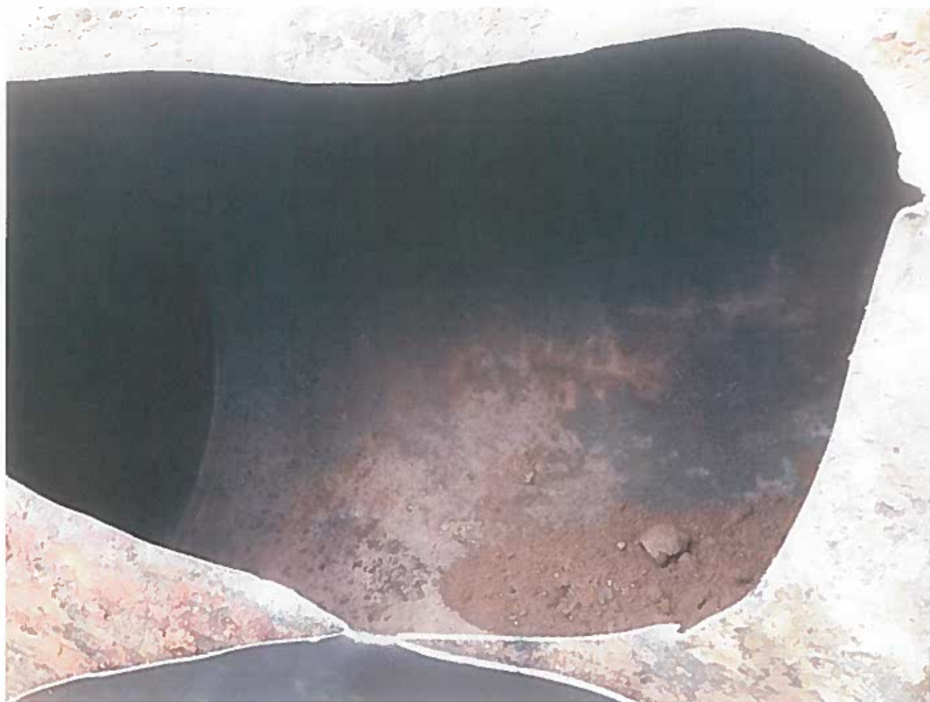
Photograph #3: Tank Cleaned out
