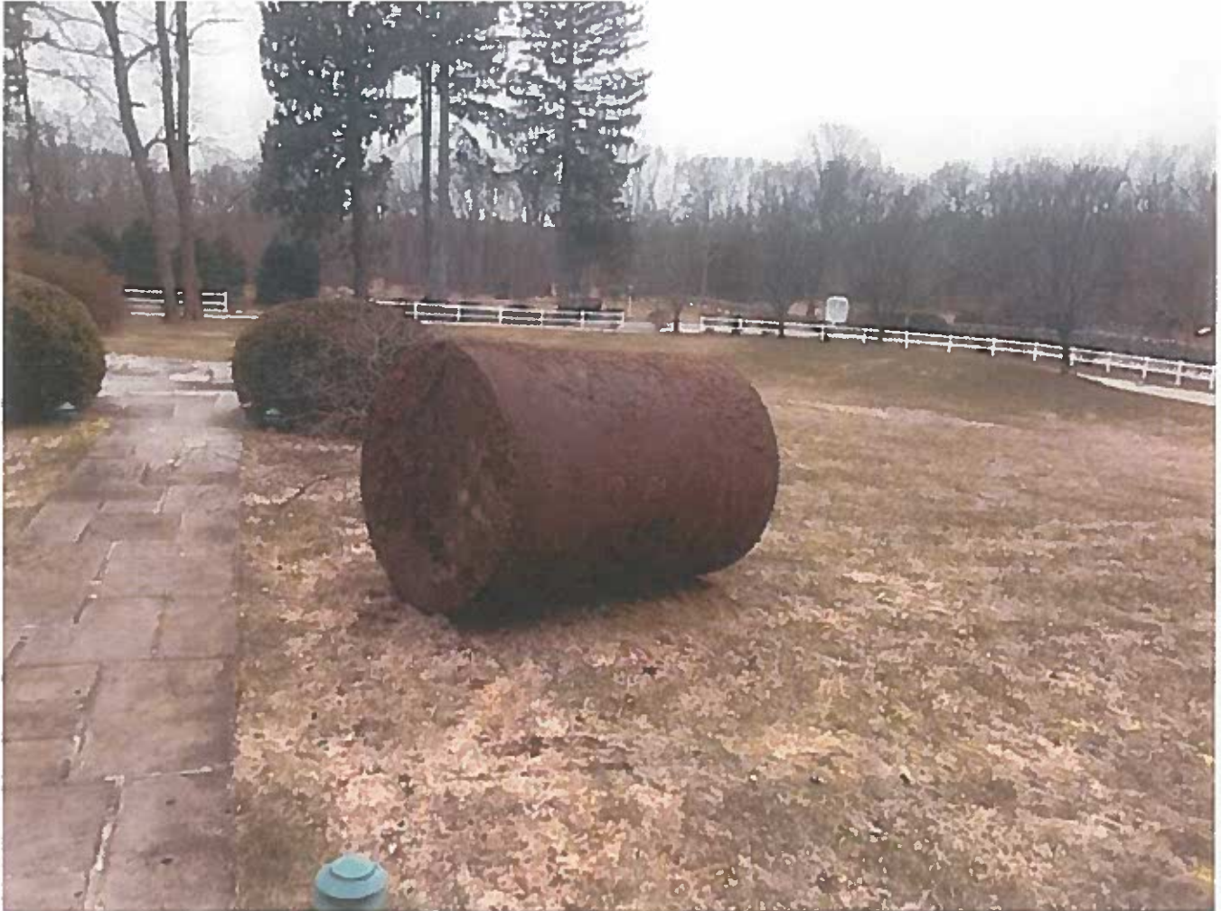
Photograph 2: 550 UST out of ground
